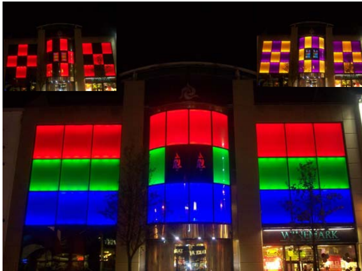
Left: Installation of Tryka Strip Module 36s at the M Club, Belfast. Installation by PSD Electronics. Pictures courtesy of Wine Inns PLC.
